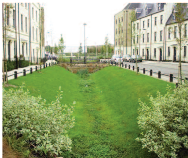
Figure 12.13: Swales at Upton, Northampton, UK
